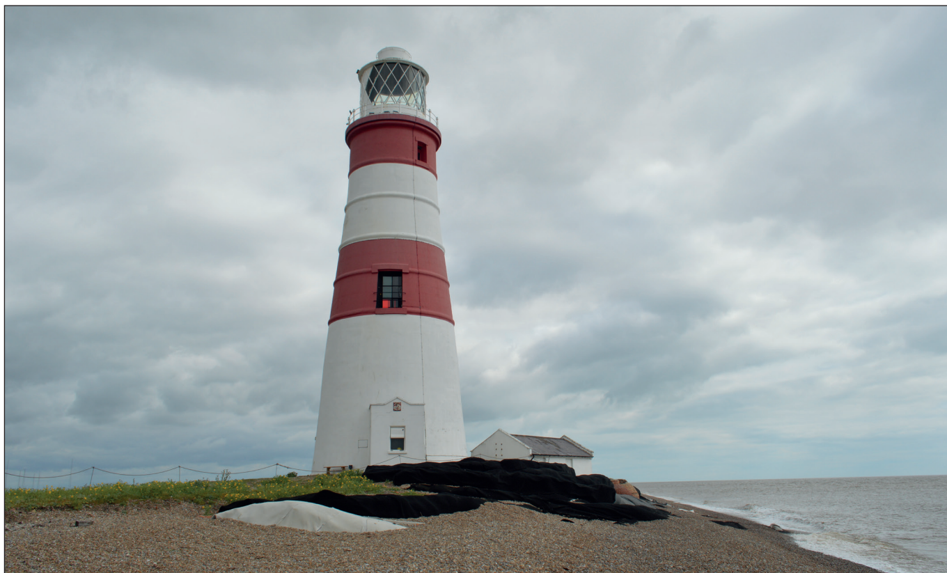
ABOVE: The final lighthouse that existed at Orfordness in 2017 before it gave way to the encroaching sea. Attempts to preserve the structure by slowing the rate of erosion with black rubber mats along the shore eventually proved inadequate. Decommissioned in 2013, the structure was finally demolished in the summer of 2020.
