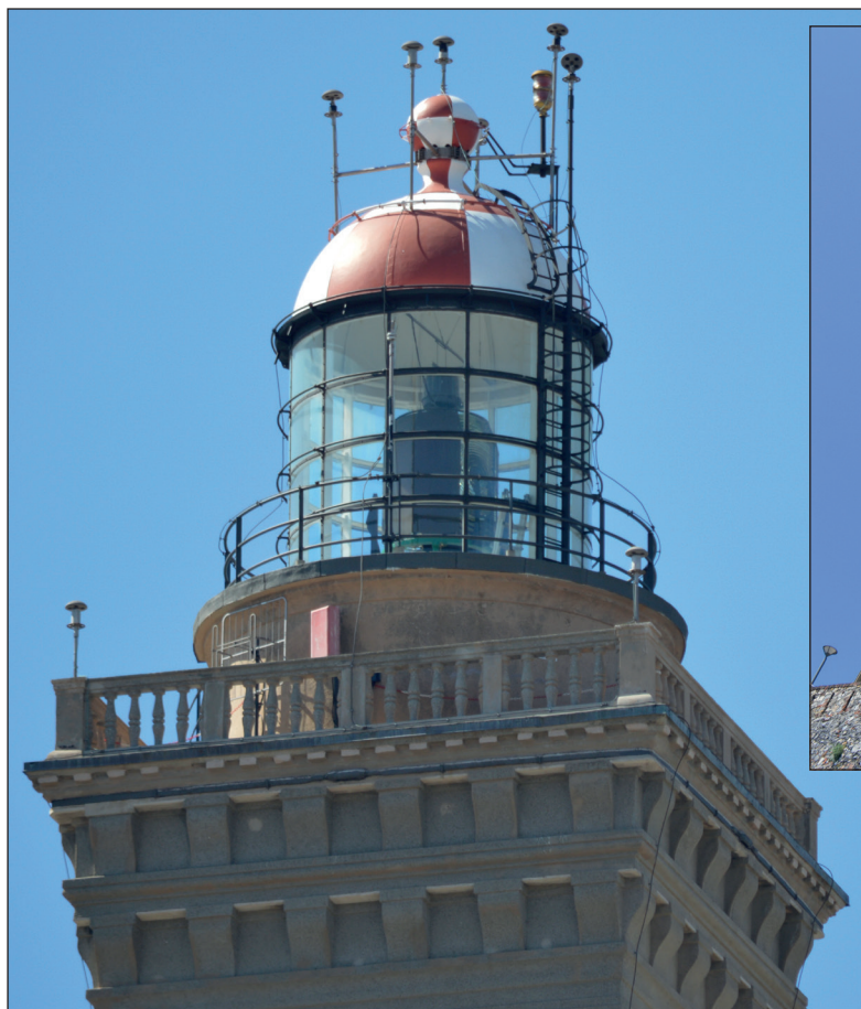
LEFT: The modern lantern with its 20th century electric apparatus.
