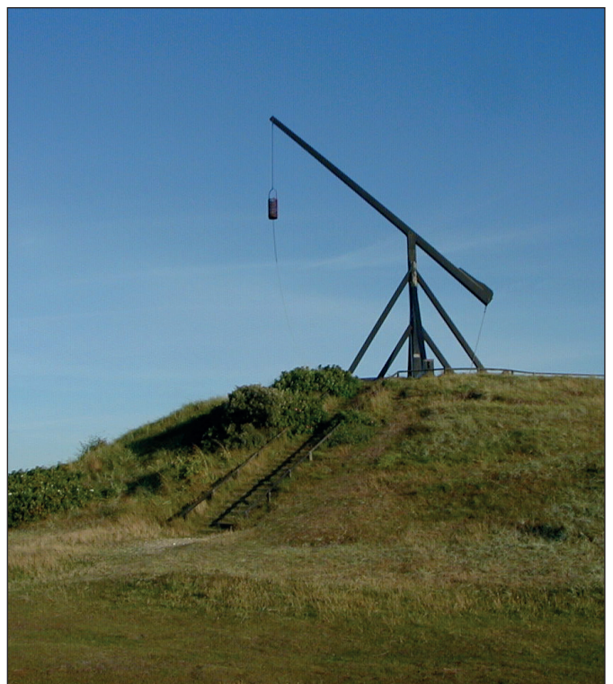
ABOVE: An example of a swape light or vippefyr, is located at Skagen in Denmark. Made of wooden beams, the design was based on a simple lever mechanism to elevate a brazier burning wood or coal (if it was available) to sufficient height for it to be seen by navigators.
