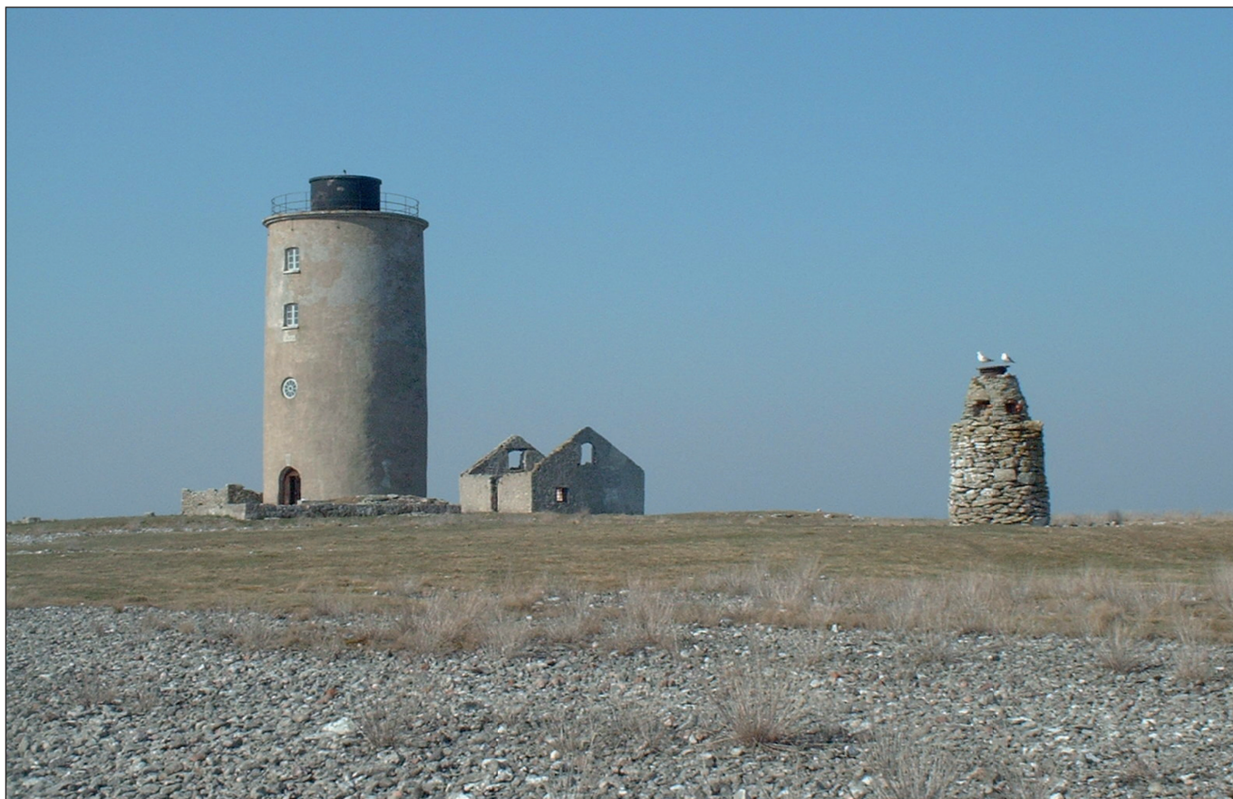
ABOVE: On the small island of Ostergarnsholmen are some remains of efforts in earlier centuries to provide lights at night. The flat-topped cylindrical stone tower is typical of an early fire tower. BELOW: Landsort, Sweden (1651).
